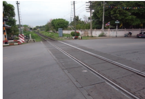
Figure6: Concrete Rail Cross (The Chainarong Rail Cross).
