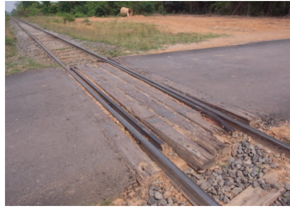
Figure4: Wooden Surface Rail Cross (the Nong Pet Nam Rail Cross).
