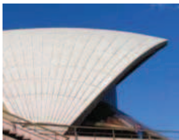
Figure 15. Glazed white granite roofs.
