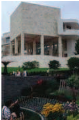
Figure 10. View of a building showing the usage of travertine.
