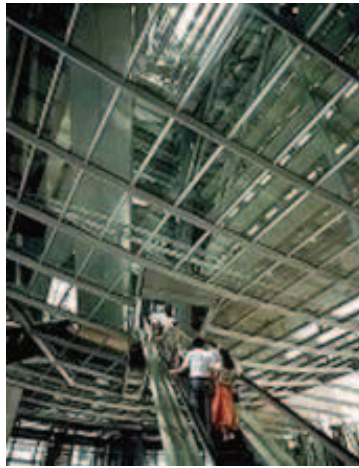
Figure 3. Escalators that rise up through a glass “underbelly”.
