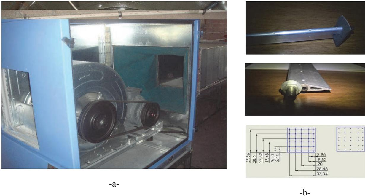
**Figure 2.** A-Cell type aspirator and its interior; B- averaging pitot tubes and distribution of measurement points.
