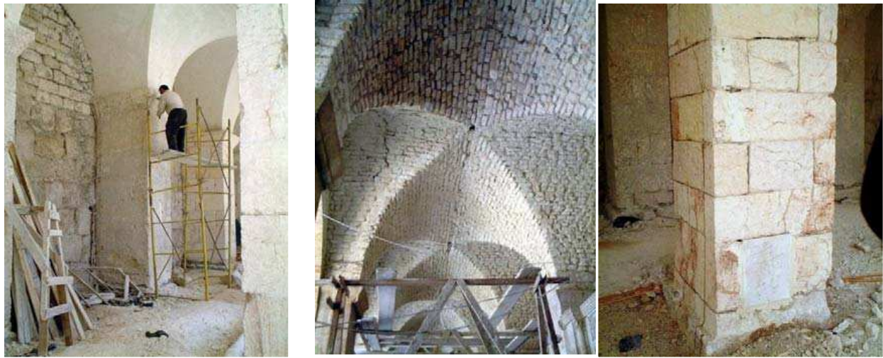
Figure 35 The restoration of pillars, walls, and cross vaults (Restoration committee 2002).
