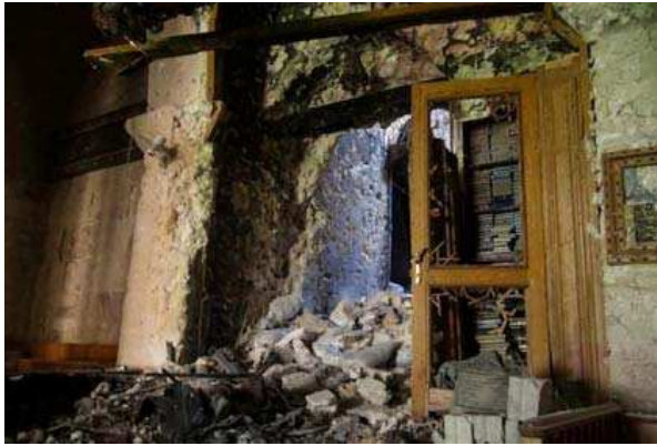
Figure 49 The southern gate (APSA 2013)
