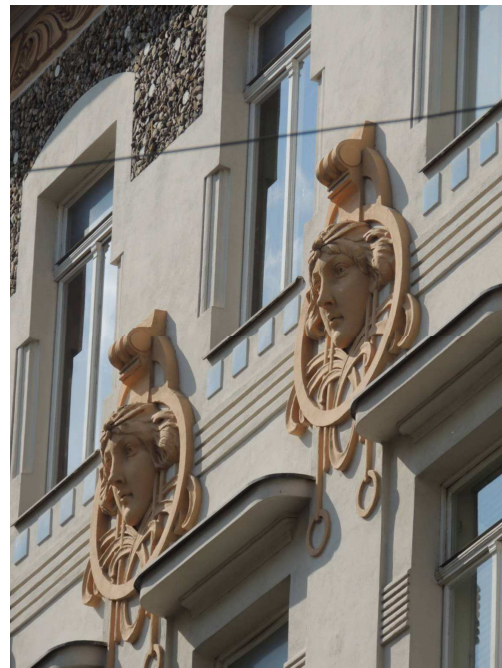
Ill. 4. Town house located at 3, Mohsgasse (design by Moritz O. Kuntschink, 1903/1904), Vienna
