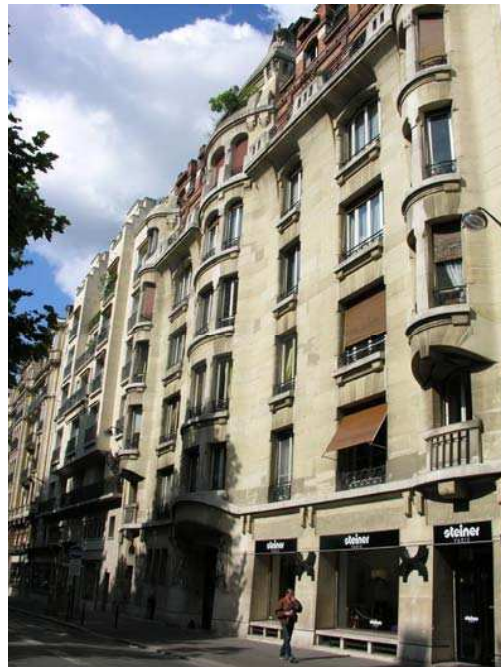
Ill. 6 The Bon Courage house located at 67, Boulevard Raspail (design by Léon Tissier, 1913), Paris (photo by B. Makowska, 2014)
