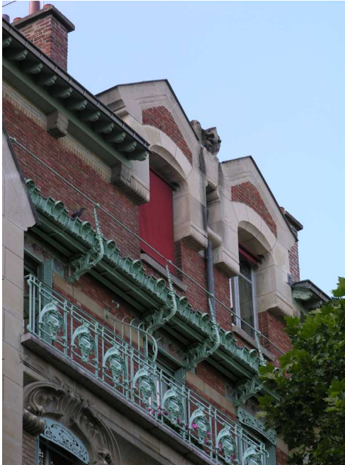
Ill. 7. The Castel Béranger house located at 14, rue de la Fontaine (design by Hector Guimard, 1894-1898), Paris (photo by B. Makowska, 2014)
